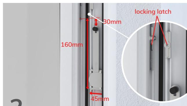
**2** Insert the blockade into the window frame at a distance of about 160 mm from the locking latch (it is important that to position the blocking arm to be approx. 30 mm under the locking bolt).
