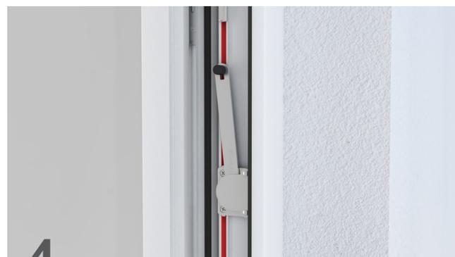
**4** Set the blockade arm in the groove axis.
